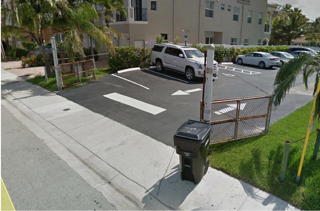
Figure 2 – Existing Gate and Fence
