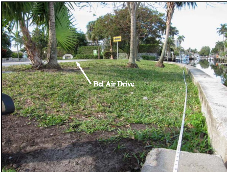
Photo 8: Upland view showing the proximity of the Bel Air Drive elevation in comparison to the existing bulkhead cap elevation.
