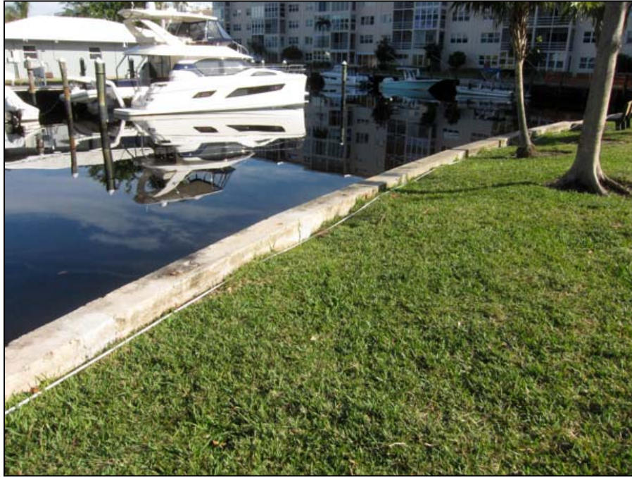
Photo 7: General view of the uplands behind the west portion of the Property bulkhead. Note intermittent depressions in the soil behind the cap.
