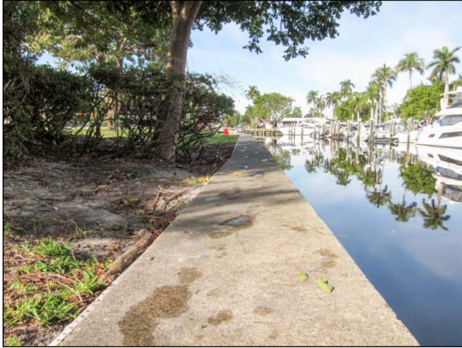
Photo 3: Overall view of the Property bulkhead looking west from Station 0+00. Note cap is sloped slightly landward.
