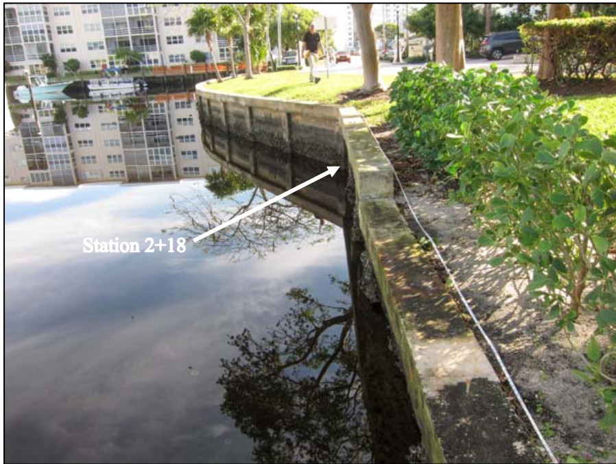
Photo 6: General view of the west end of the Property bulkhead (Station 2+18) looking east from the neighboring bulkhead.
