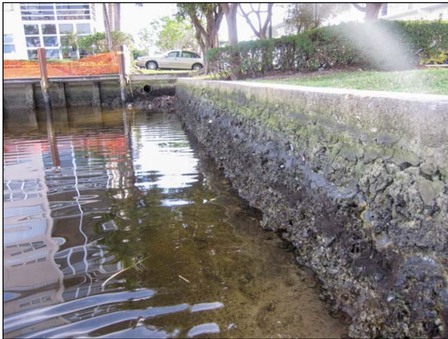
Photo 2: Overall view of the Property bulkhead looking east towards Station 0+00.
