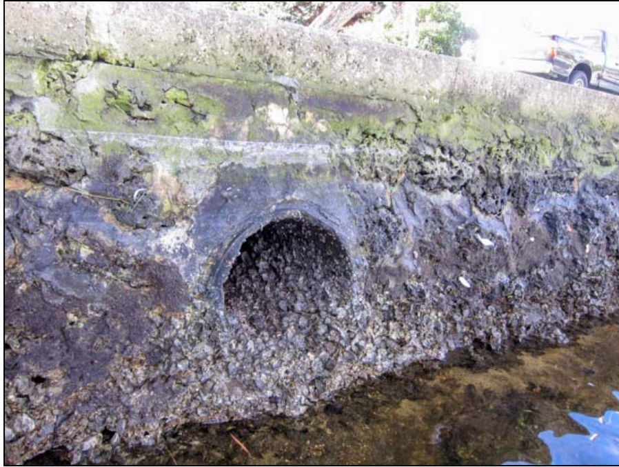
Photo 15: View of the outfall extending through the Property bulkhead at Station 0+38.
