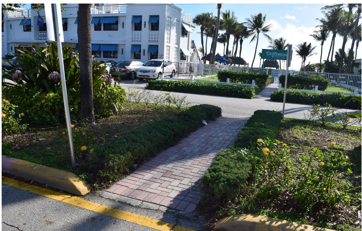
MEDIAN BREAKS and mid-block crossings are inadequately marked and inconsistently designed.
