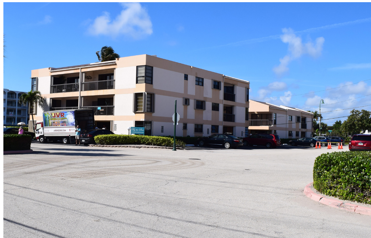
UNNECESSARILY WIDE INTERSECTIONS could be reduced with bump-outs.
