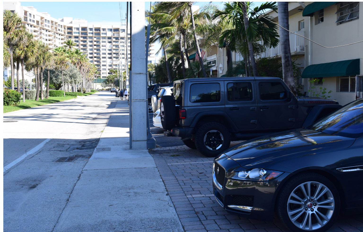
SIDEWALKS ARE TOO NARROW and are cluttered with utility poles.
