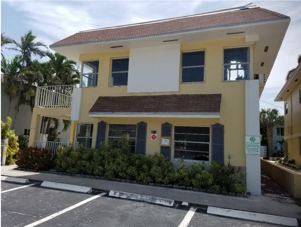
Photo 1 - East Front Wall of Building
