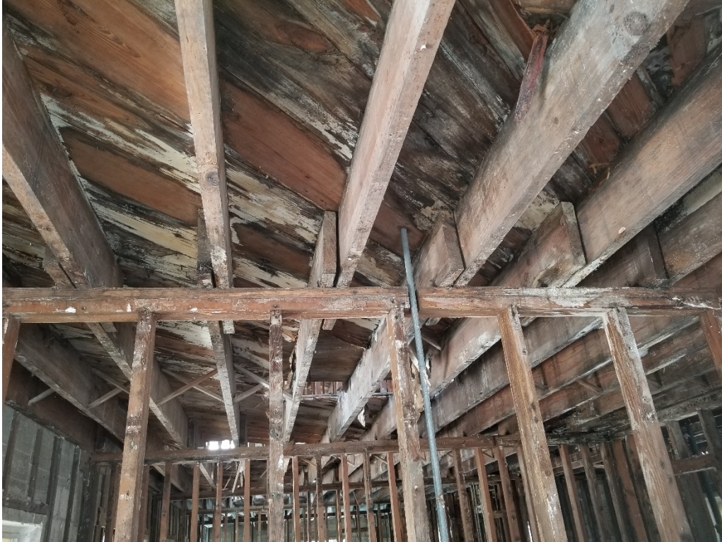
Photo 2 - Overall View of Second Floor Interior Bearing Walls and Roof Joists
