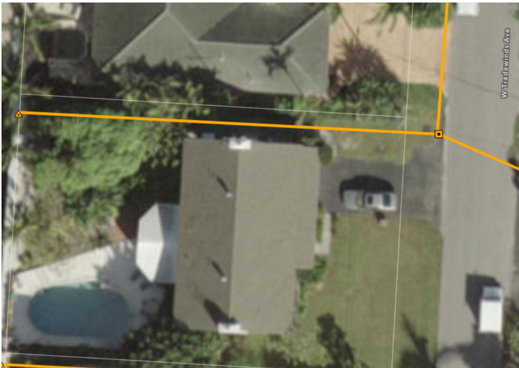
4607 W. Tradewinds Ave Storm Sewer Line
