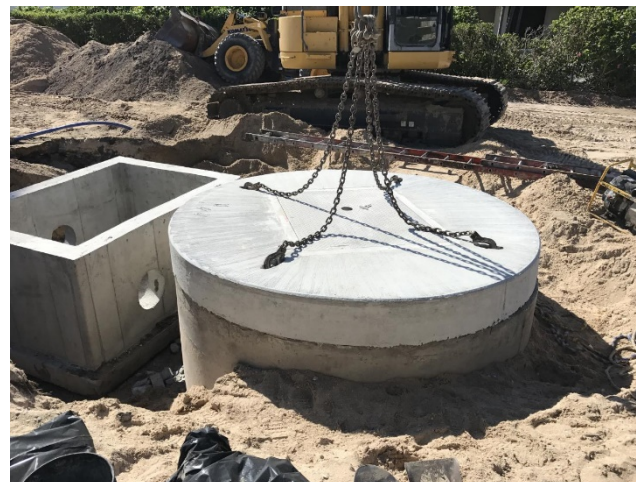
Wet Well Slab Setting
