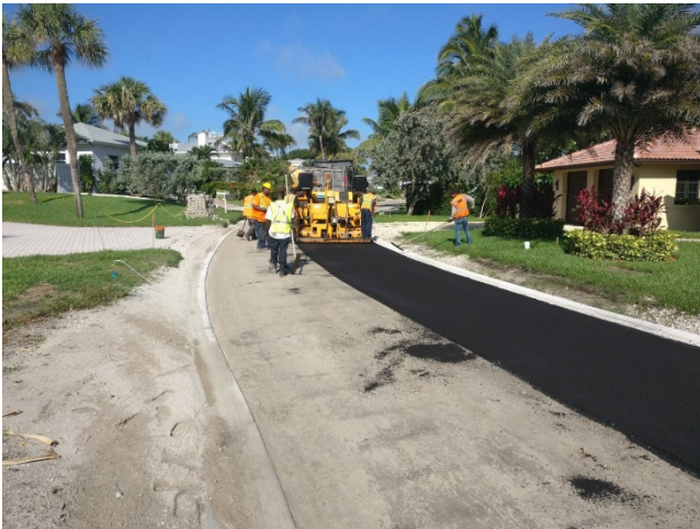
Laying Asphalt
