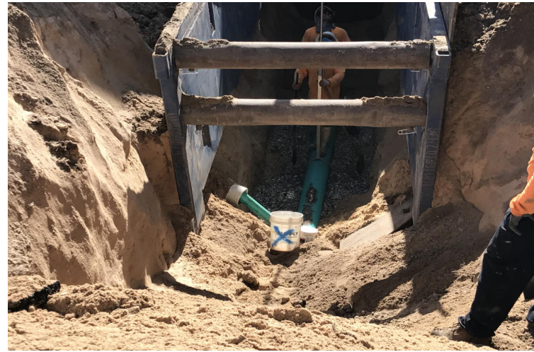
Sewer Main and Service Lateral Installation
