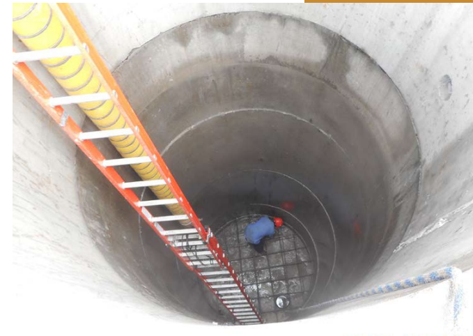
Rebar Floor Construction
