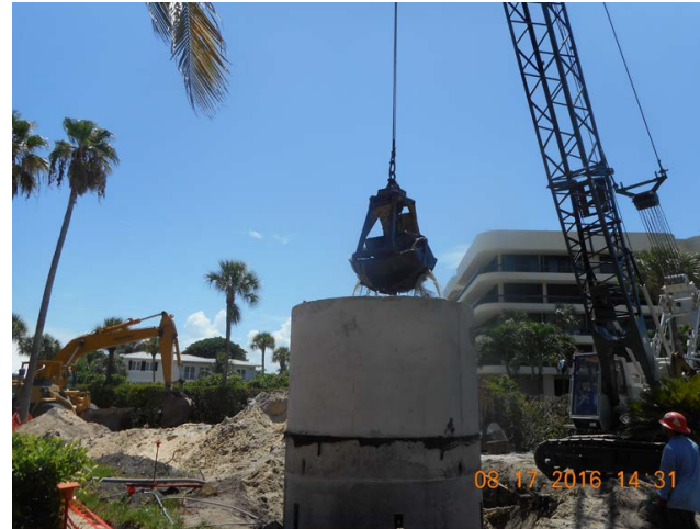
Removal of Material within Wet Well
