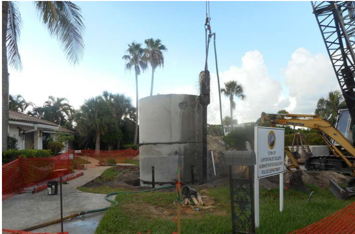
Installation via Caisson Method
