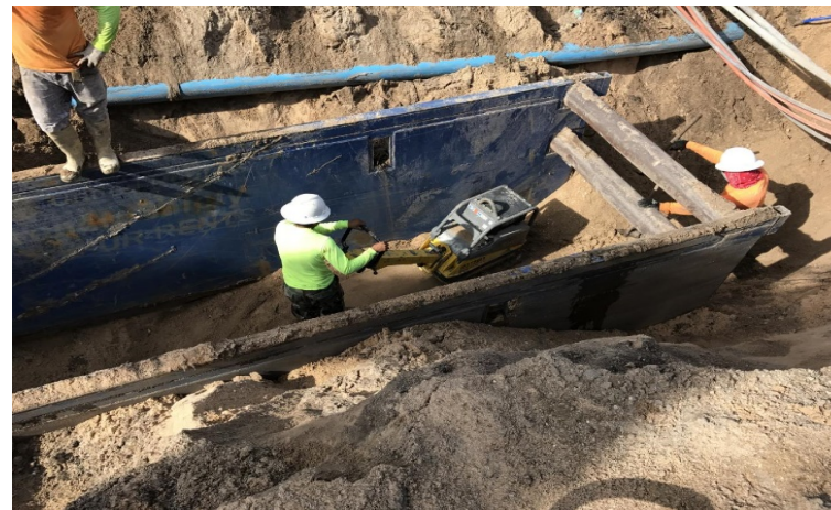
Compaction of Backfill around Pipe
