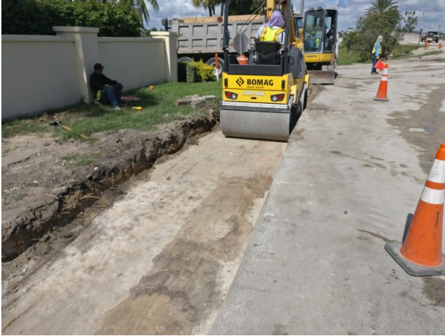
Trench Compaction
