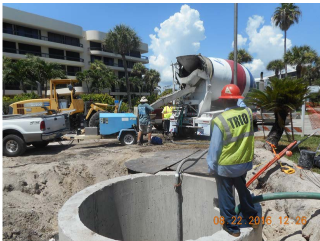
Concrete for Ballast Seal and Floor
