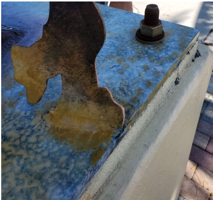
Base showing some staining from rusting mounting hardware spot loss damage to color and side edge deterioration through all levels in base areas.
