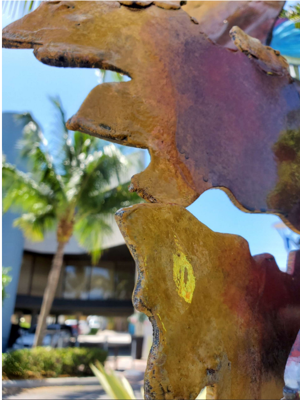
Loss of top coat paint, primer and oxidation to aluminum all visible in varying degrees in photos left edge of sculpture.
