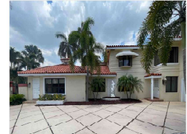
EXISTING RIGHT SIDE - EAST VIEW
