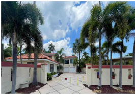
EXISTING FRONT - SOUTH VIEW
