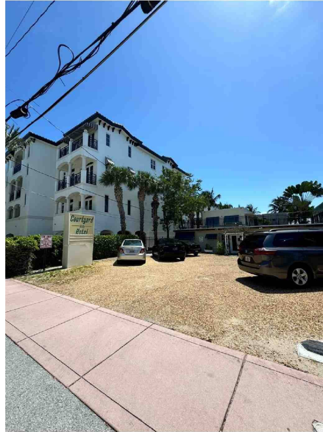
Existing Front view
