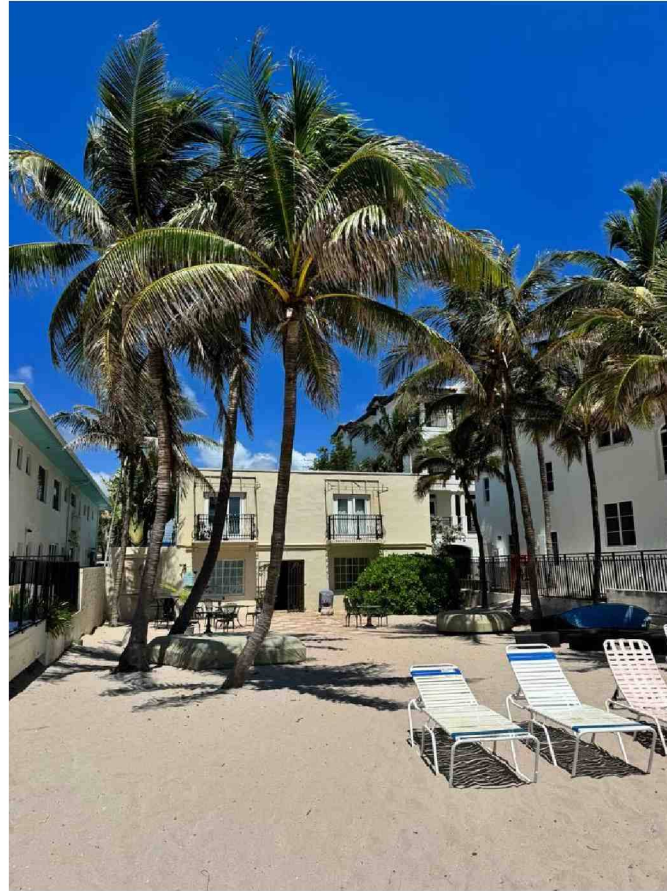
Existing Rear view
