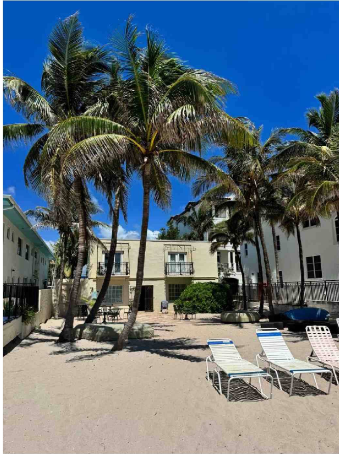
Existing Rear view
