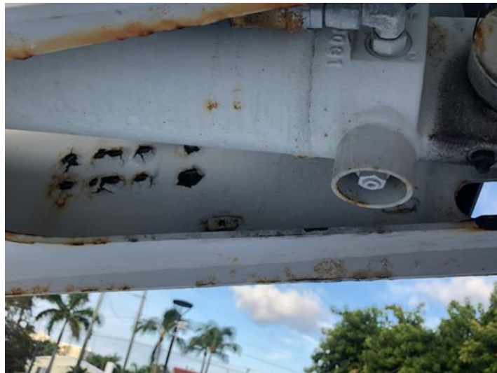
Rust on boom arm
