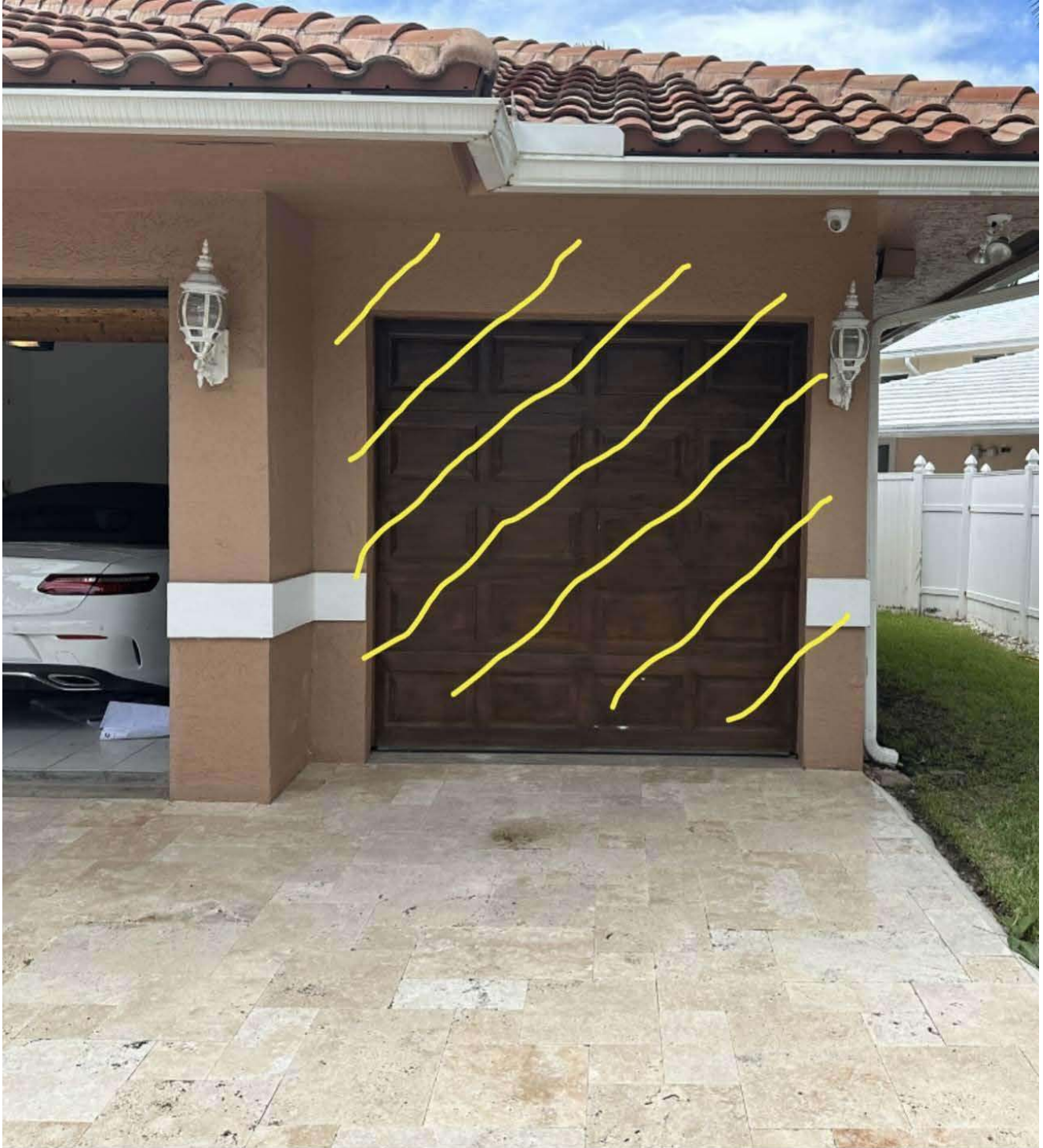
291 Imperial Lane One Car Garage Front Wall And Door Move Forward To Match The Front Wall Of Two Garage Door.
