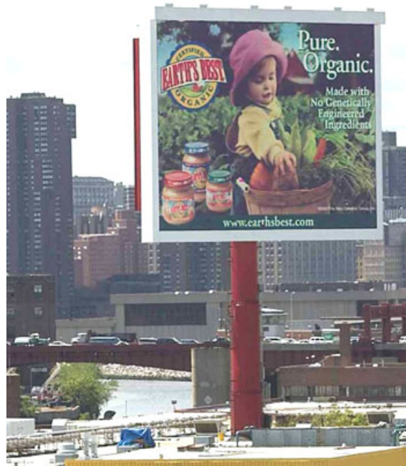
Figure 7. The world’s largest LED sign; an on-premise sign in New York City. The sign measures 90 ft tall by 65 ft wide and is mounted on a 165 ft tall steel post on the roof of building.
