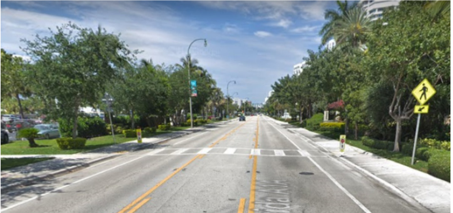
Unsignalized A1A midblock crossing (Approximately 1800 A1A)
