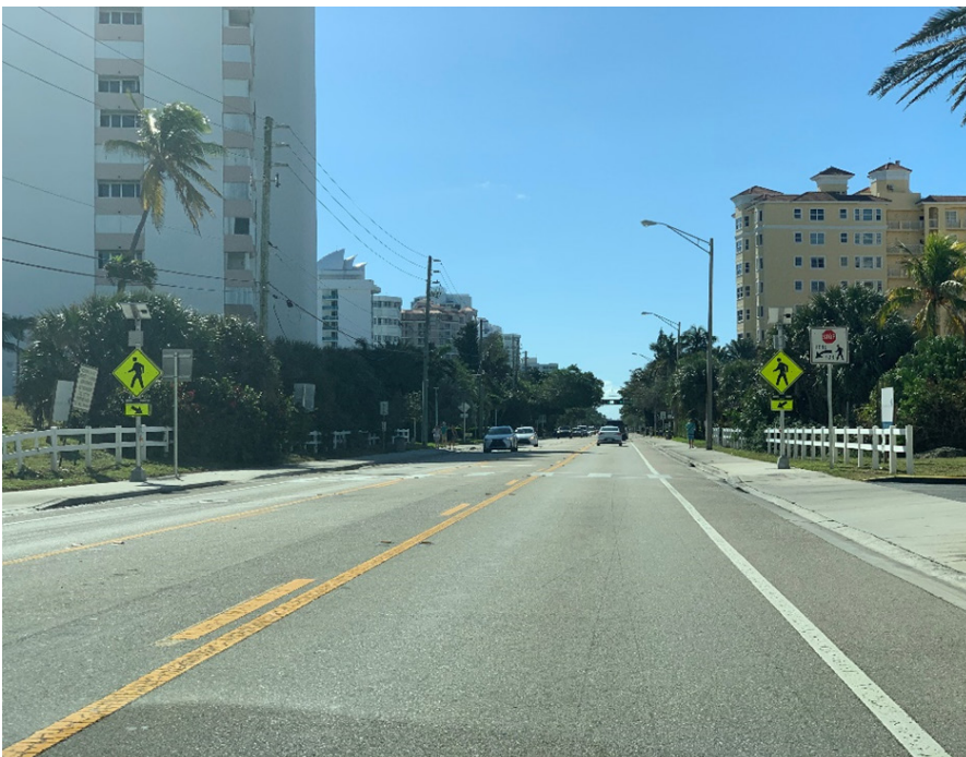
Midblock crossing with solar rapid flashing beacon
