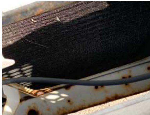
Light to Moderate Rusting Adjacent to the Radiator in the Engine Compartment
