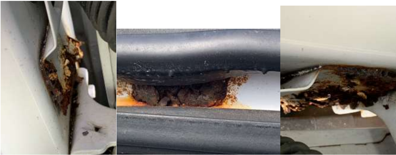
Severe Rust Noted in Several Locations on the Vehicle Cab
